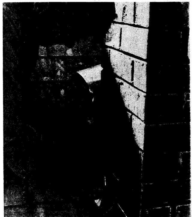
Fig. 19. Metal flashing is inserted to prevent water leaks around chimney.
