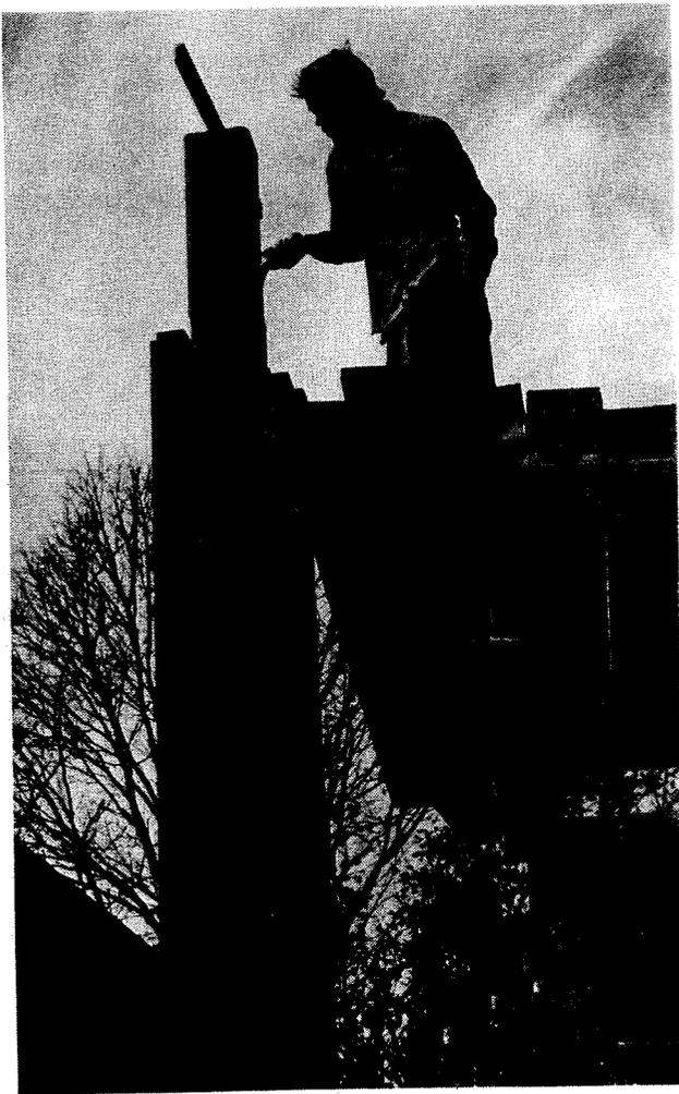
Fig. 12. Flue liner is placed first and the bricks laid around it.
