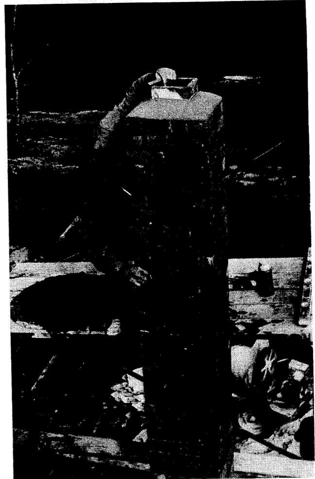
Fig. 21. Tooling the final mortar joints after topping out the chimney.
