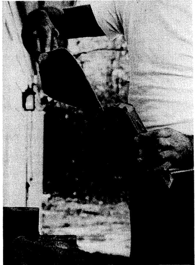
Fig. 11. Completely buttering end of chimney brick.
