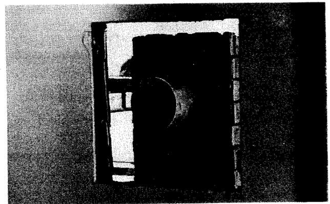
Fig. 15. Interior view, showing wall opening and thimble before bricking-in.
