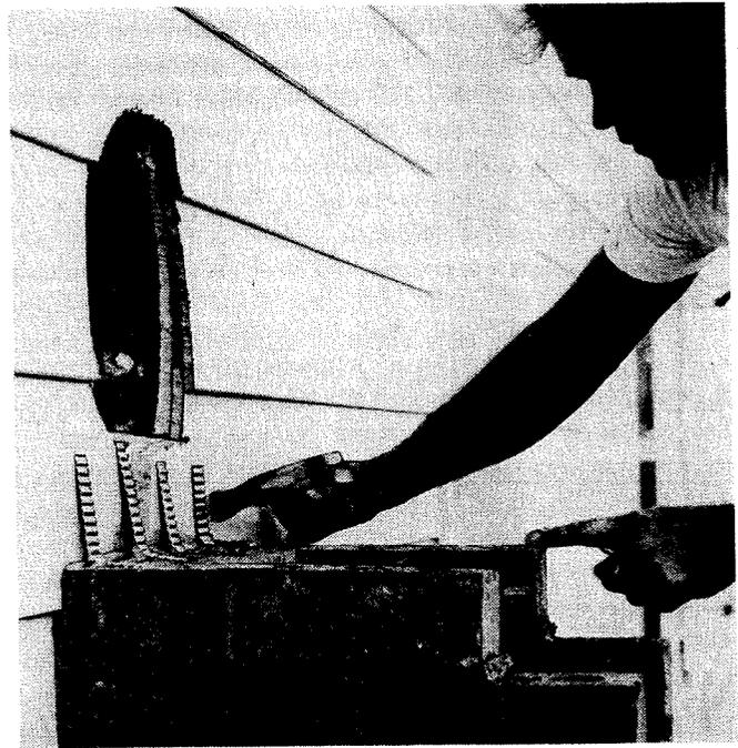
Fig. 14. Corrugated steel wall ties placed every sixth course of brick.
